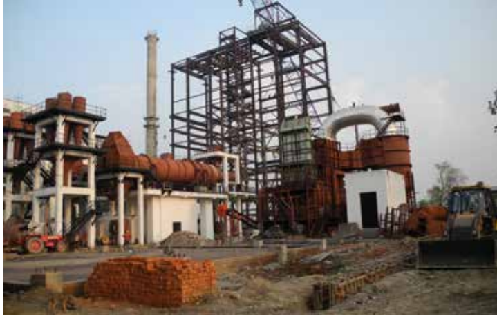
A cement plant under construction.
