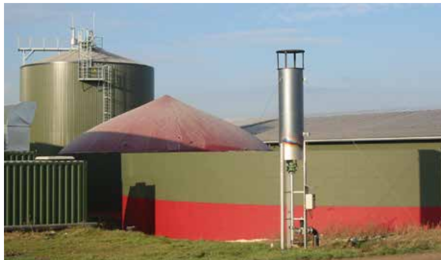
Gas flares safely release excess pressure.
